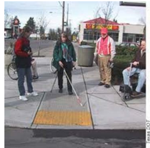
Figure 9. ADA Accessible Curb Ramp
